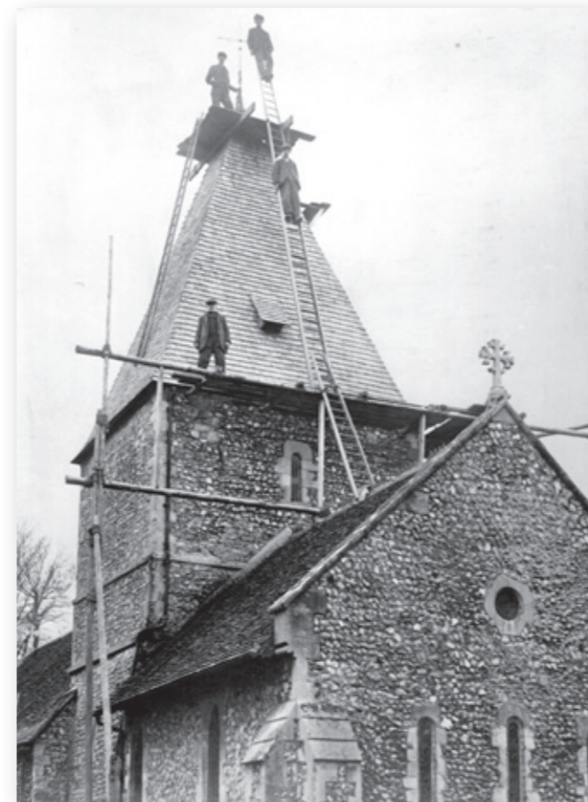
Re-shingling the spire of Iford Church in 1929 in the days before 'Health & Safety' had been invented.
